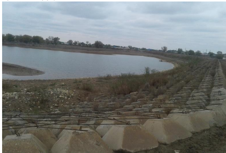
Figure 2. Laying tetrahedral on the banks of the reservoir
