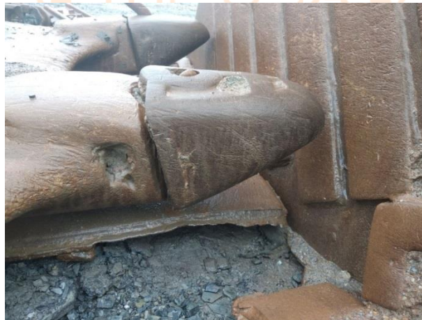
Figure 1. Defective part of HITACHI EX-1200 excavator bucket connected with cutting element and adapter part
