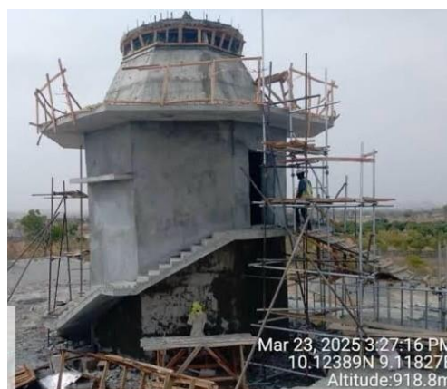
Figur 2: VLBI tower under construction at CGG Toro
