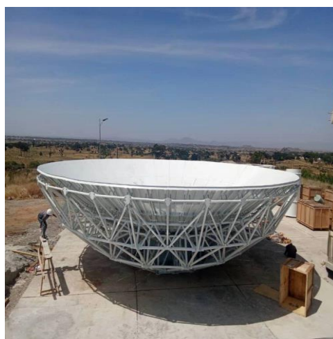
Figure 3: A 13m diameter Antenna under construction at CGG Toro
