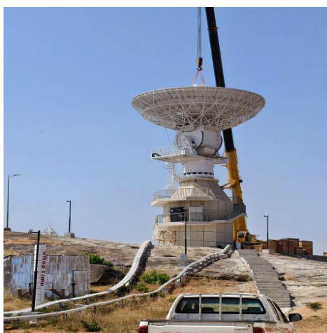
Figure 4: Hoisting of the Antenna in process at CGG Toro
