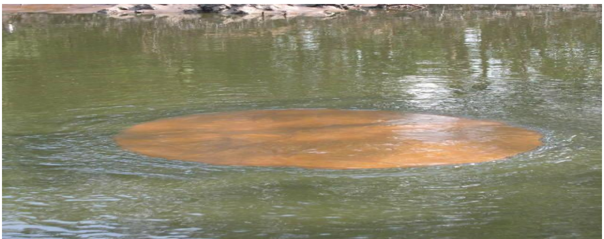
Figure 8: Leaking Underwater Pipeline.
