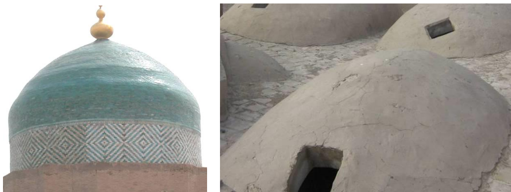
Figure 7. Spherical dome forms used for roofing the vertical dome and madrassas in the inner part of the Pahlavon Mahmud Complex
